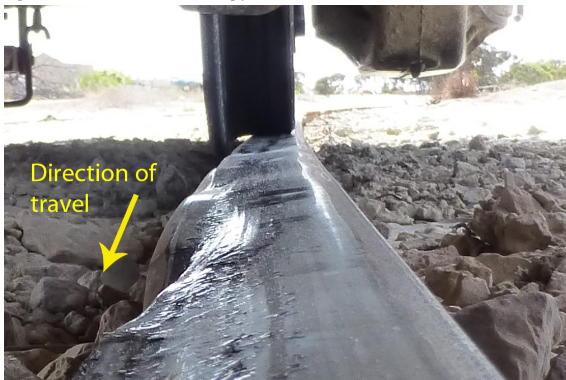
Figure 6: Rail condition and running position of wheels
