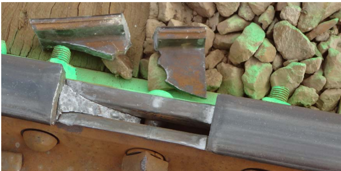
Figure 8: Rail defect in mechanical joint
